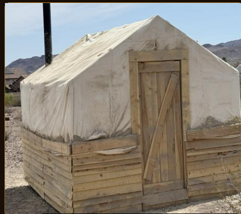
Tent house exterior — built from scratch, donated to Clark County Museum
